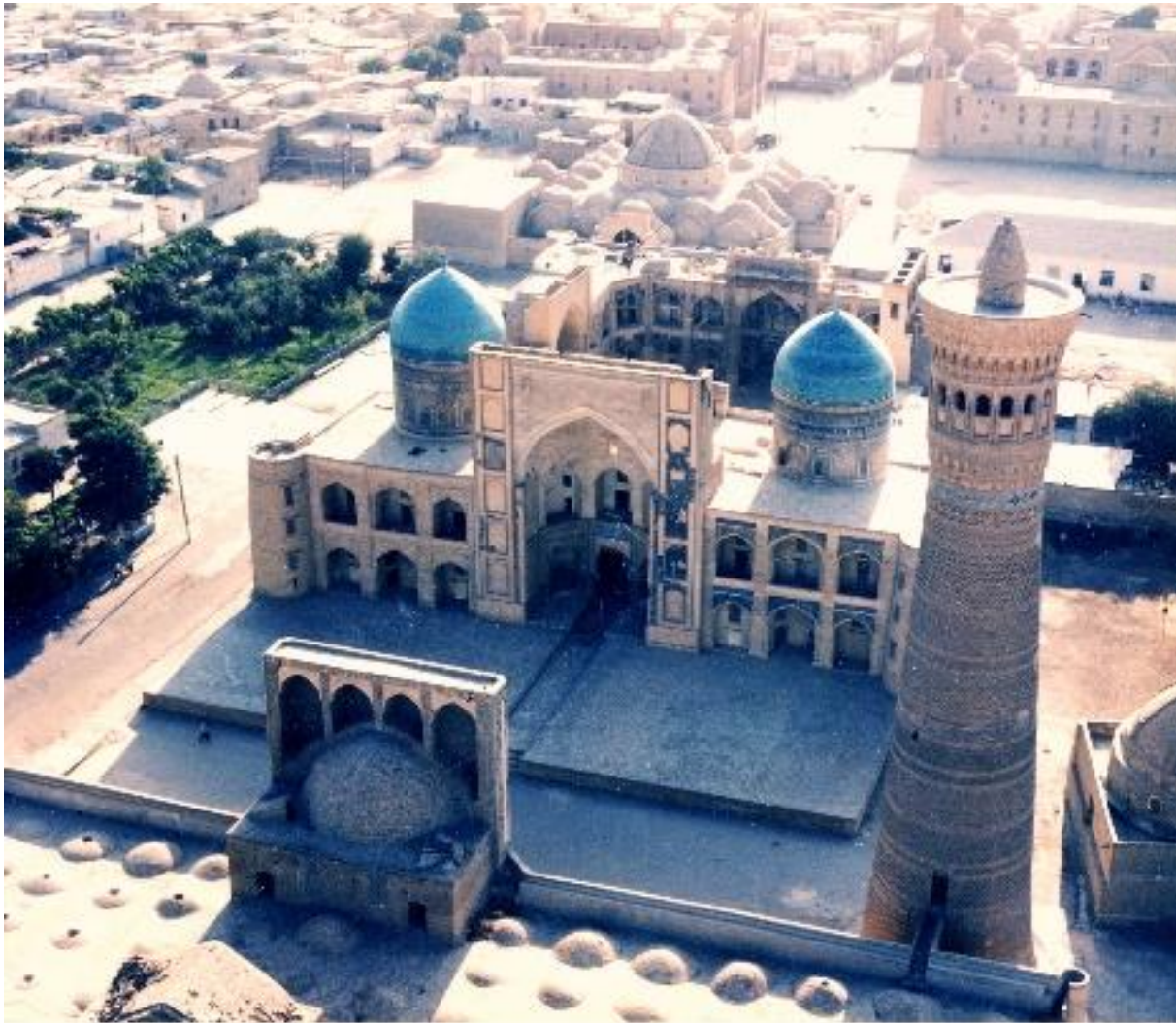
Figure 9. Ensemble Pa-i Kalyan. 12 th -15 th -16 th centuries. View from above (Archive Glav NPU, photo 1980s).
