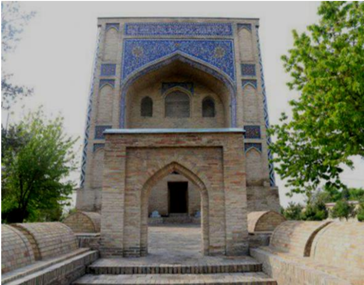
Figure 34. The stepped corridor with brick graves on both sides rises 170 cm and reaches the entrance of Abubakr Kaffal ash-Shashi Tomb. The arch order is in Iranian form. (2022)
